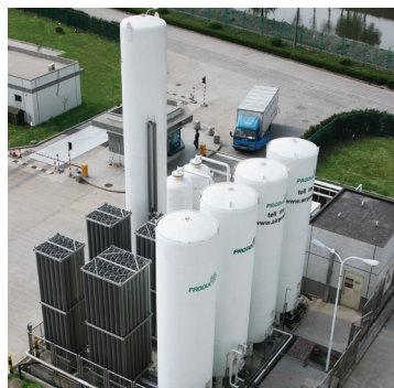
▲ Figure 1. Nitrogen users can choose from a range of options for on-site nitrogen production to meet a variety of needs, including cryogenic air separation, pressure swing adsorption, and membrane systems (left to right).
